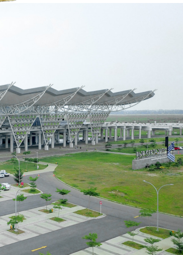
Bangunan Terminal Terminal Building
